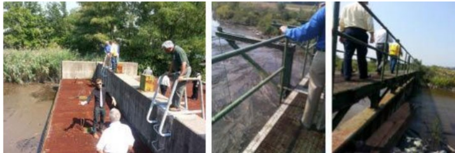
Figure 4-1: Physical Inspection of Existing Risk Reduction Infrastructure. Teams assigned by the New Jersey Department of Environmental Protection have endeavored to catalogue Superstorm Sandy’s impact on berms, tidal gates, and other existing risk-reduction infrastructure. Physical inspection is a key part of the State’s assessment of the current condition of measures to identify necessary repairs as well as opportunities to enhance existing measures to address future extreme weather events and maximize federal investment.
